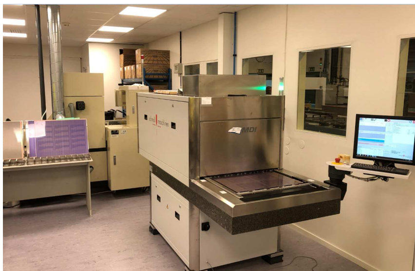
Schmolz MDI direct imaging installed in our new cleanroom in our Swedish factory.
